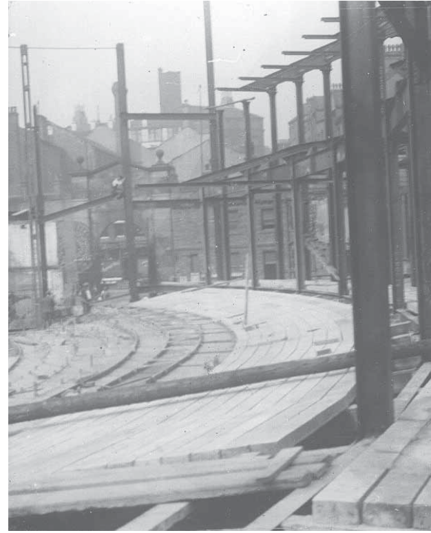
Frame, cantilevered tiers and lightweight infill planks
