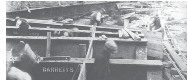
Cantilevering over the Beck
