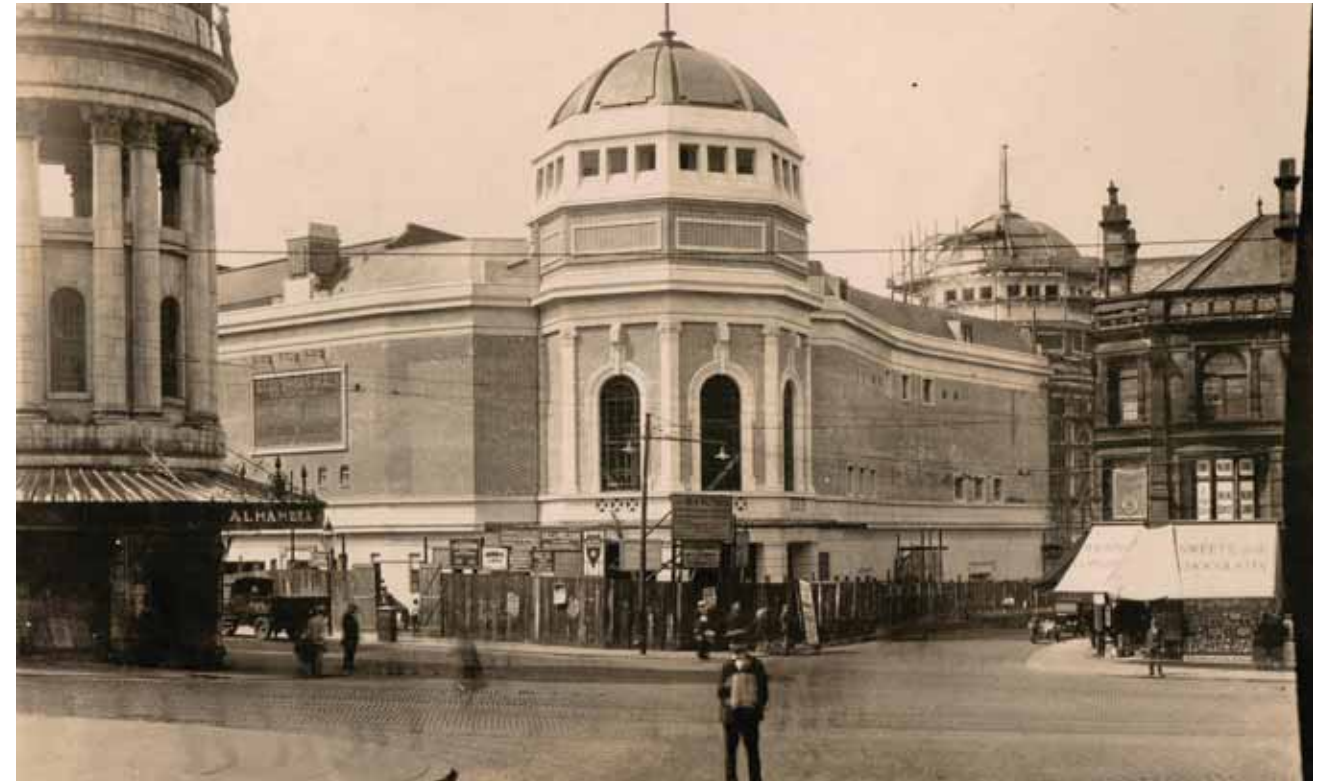
New Victoria nearing completion and highlighting prominence of corners and width of Godwin/Brewery Street
