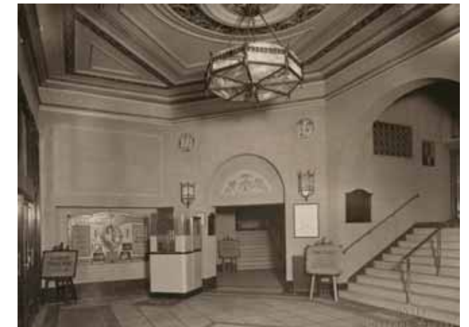
Entrance lobby within the north turret
