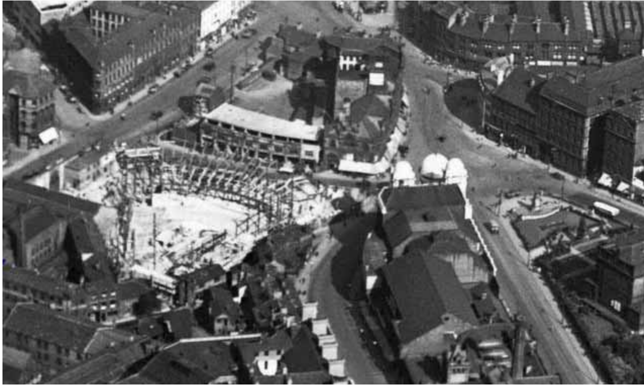
Ground floor slab and steel frame underway in 1929
