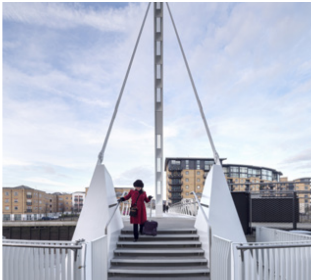
Greenwich Reach Swing Bridge © Photography by Simon Kennedy
