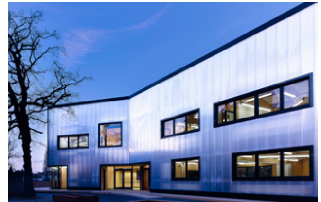
Graveney School Sixth Form Block (Bradford Building)
