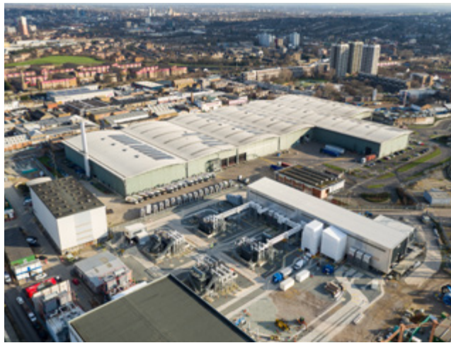
Southwark Integrated Waste Management Facility
