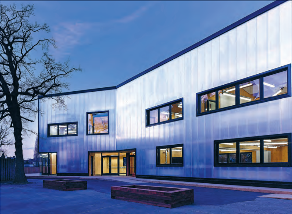
Graveney School Sixth Form Block (Bradford Building)
