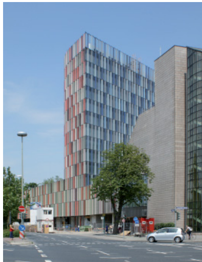
offices for the KfW banking group, frankfurt
